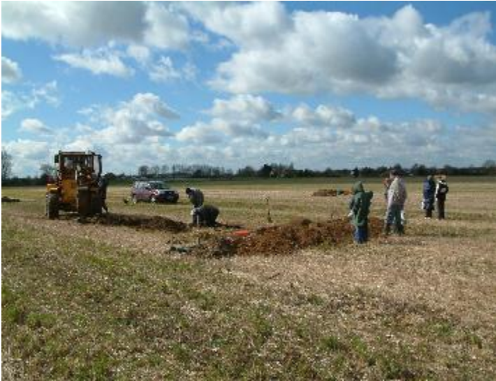
Fig. 7: In goes Trench E.
